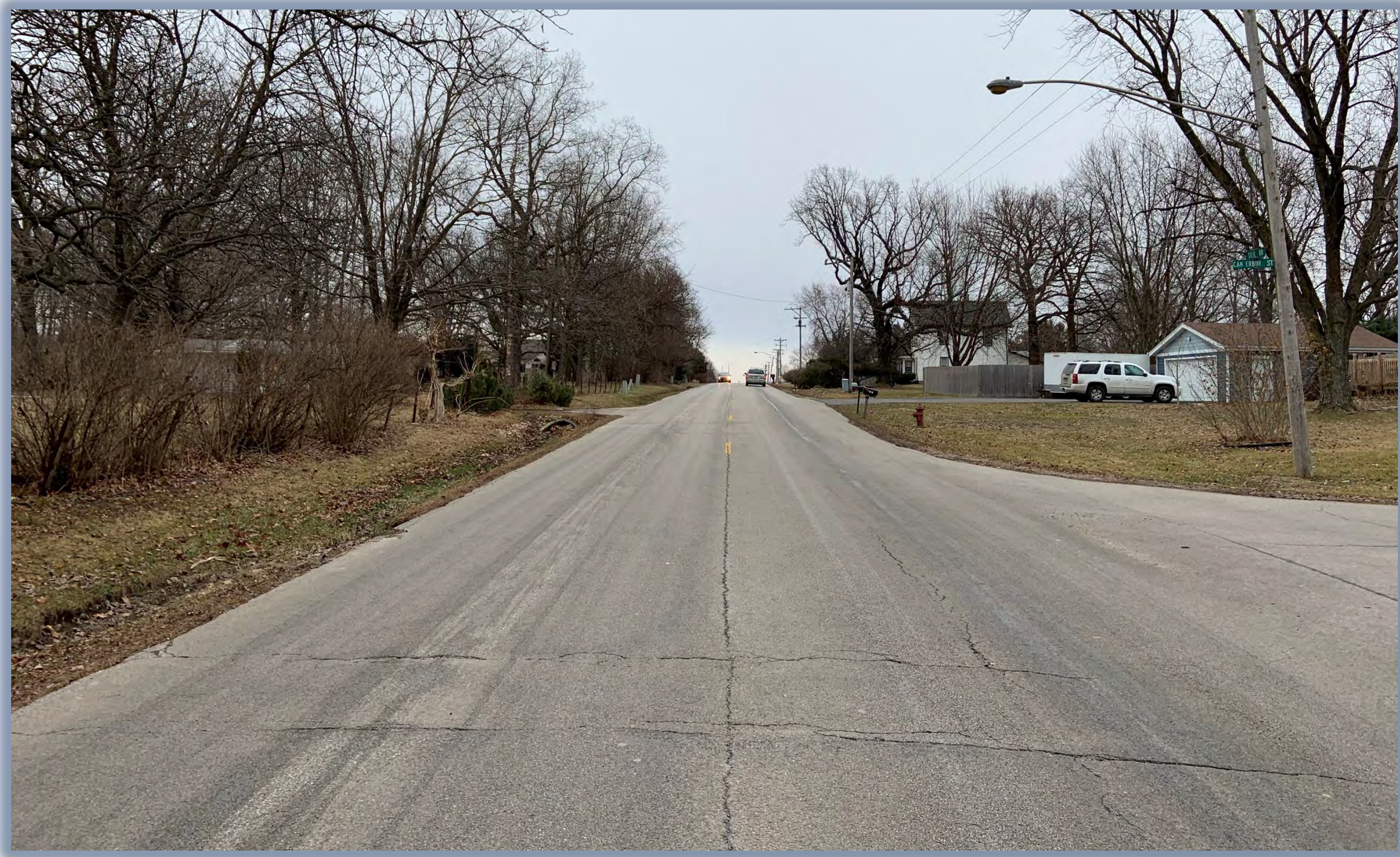
EXISTING CONDITIONS LOOKING EAST
