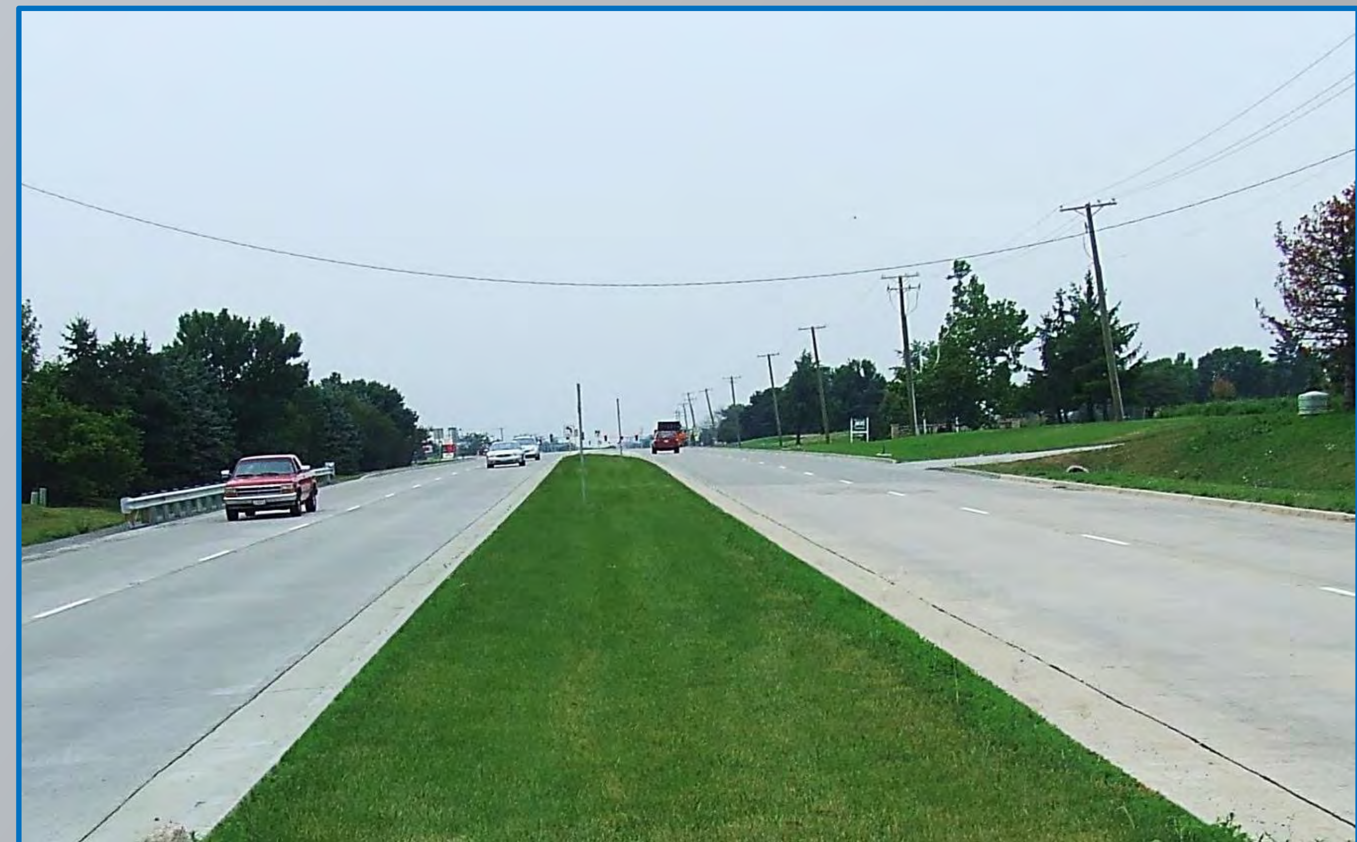
Example of a Landscaped Barrier Median
